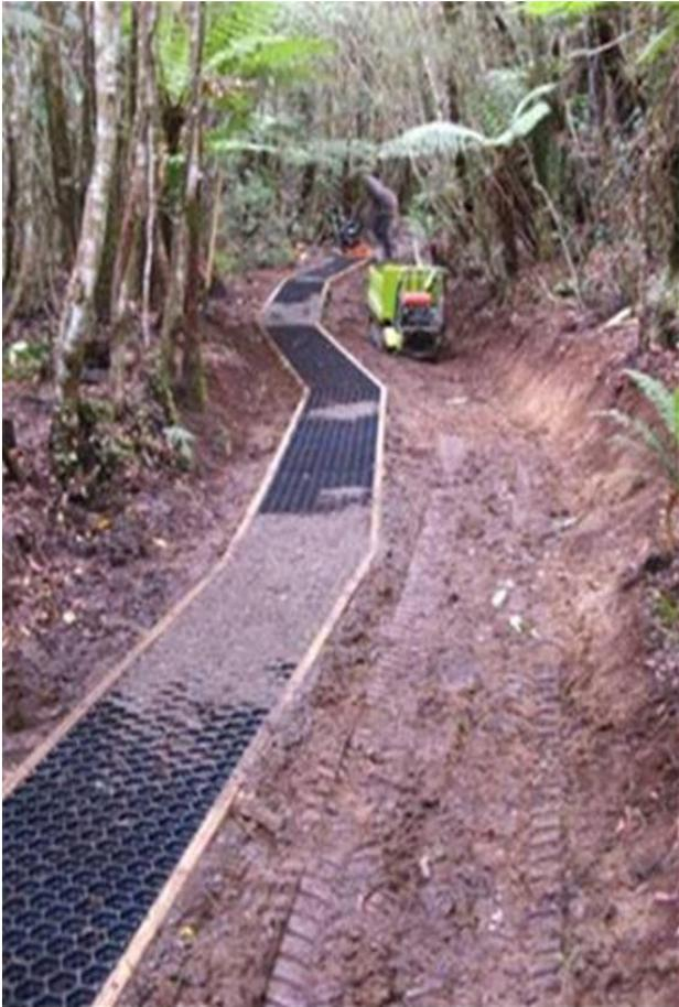
Photos. (Left): 'Presto' Geoweb based system used to stabilise BAM on walking tracks. (Right): 'Jakmat' Geocell system being used to stabilise aggregate walking track surfacing (Photos courtesy of T. Butler, Frame Group Ltd).
